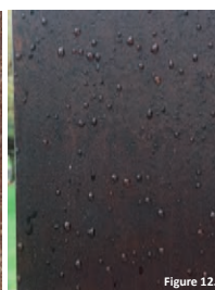
Conservation of works: Figure 11. Detail of a Corten steel work before restoration, with a dirty surface and limescale residues. Figure 12. Cleaning of the surface and application of protective coatings, to protect against excess moisture. Figure 13. Students from the Degree in Heritage Conservation, on learning practices for the works restoration.
